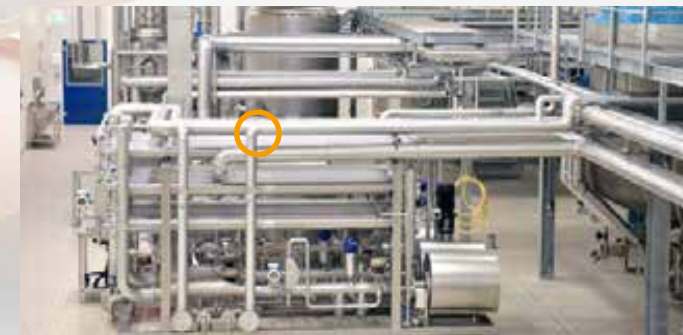
Inspecting of weld seams in stainless steel pipes
